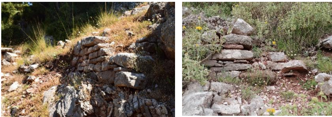
Image 1-5 and Image 1-6. Foundations of buildings in the "Tsouknides" location of Agios Georgios hill. Source: NTUA Research Team, 2023.
