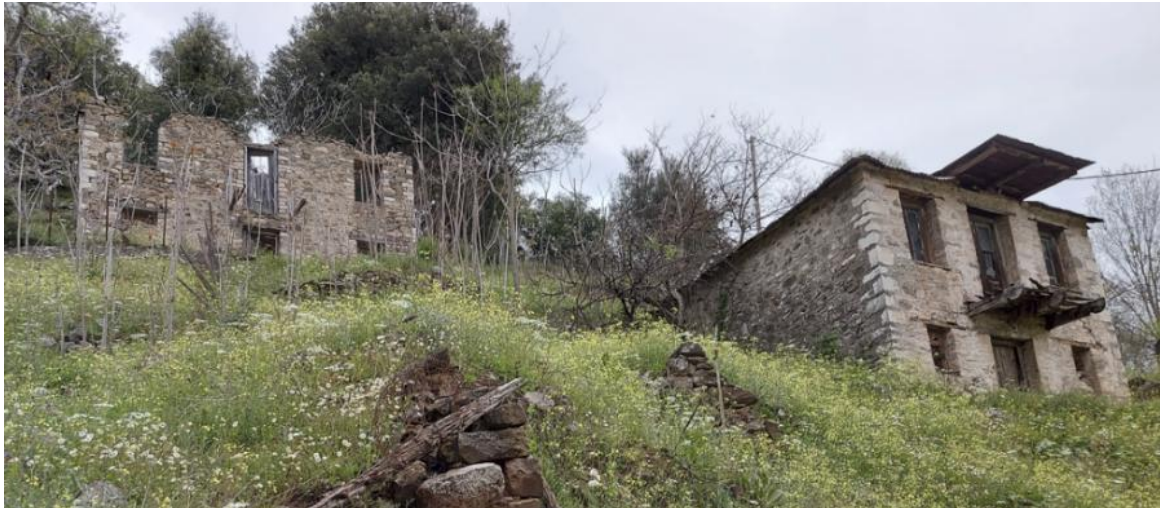
Image 3-48. Abandoned buildings. Source: NTUA Research Team, 2023.
