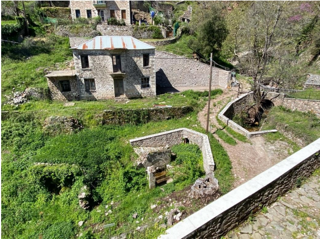
Image 5-22. The fountain, where the "kazanaria" were once located in the center of the settlement, and in the foreground behind it, the two-story building with the former "Switzerland" cafe on the ground floor and the residence of the Alatari family on the first floor. To the right in the stream there was also a ground-floor tavern-grill which was destroyed in a flood around 1990. Source: NTUA Research Team, 2023.
