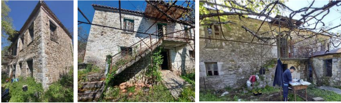
Image 3-26. Two-story building -Karageorgou House- (left), half-story building with external staircase (center), two-story building with external staircase (right-House "of the Teacher"). Source: NTUA Research Team, 2023.
