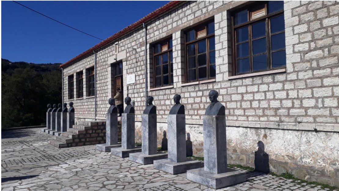
Image 3-17. Southern view of the Viniani Elementary School with the busts of the ministers of the "Mountain Government". Source: NTUA Research Team, 2023.
