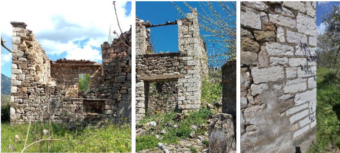
Image 3-32. Building corners reinforced with a larger surface of stones with carved faces. Source: NTUA Research Team, 2023.
