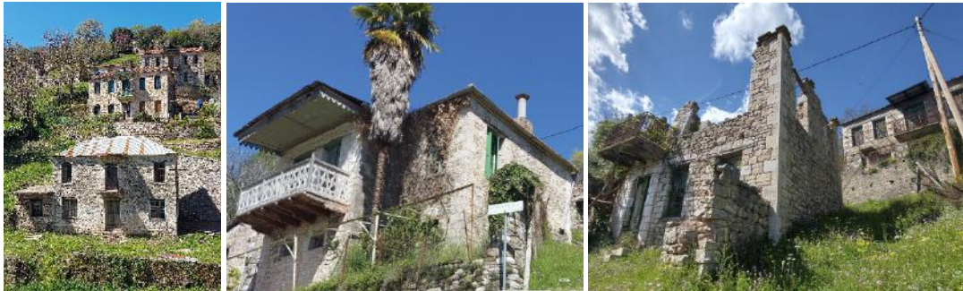
Image 3-9. Two-story and semi-detached buildings in Viniani. Source: NTUA Research Team, 2023.
