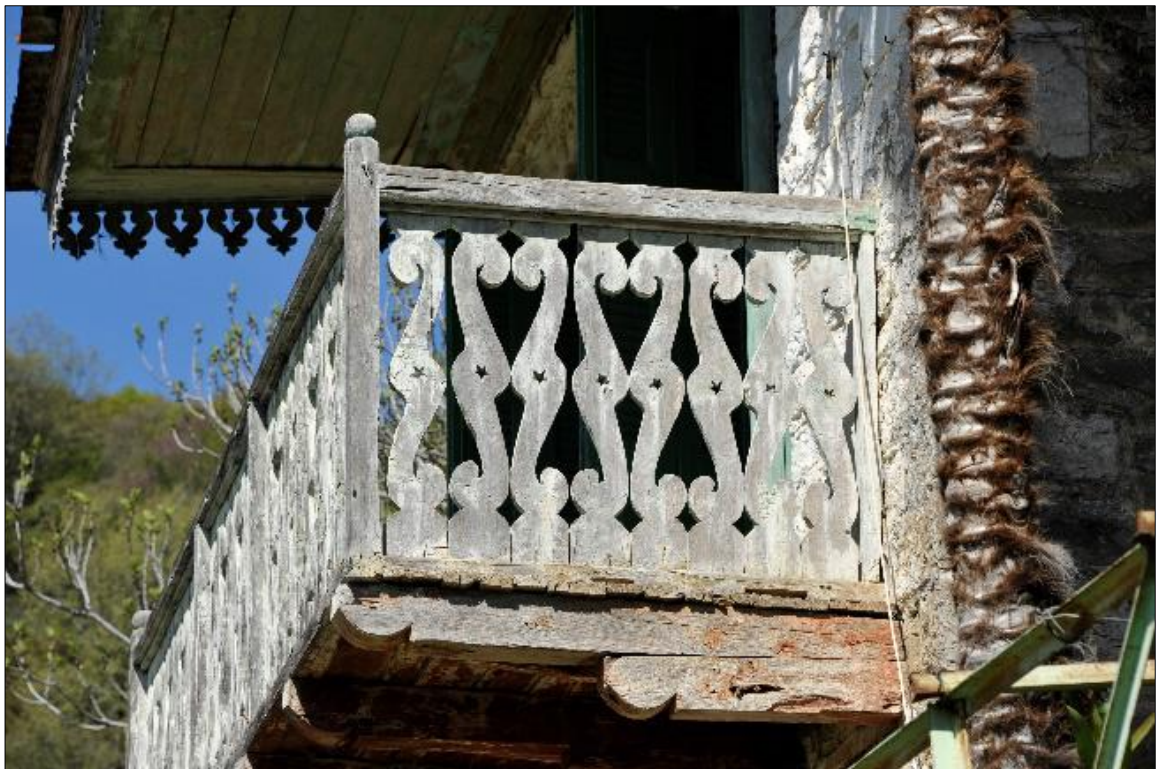
Image 3-12. Wooden railings and hanging stalactites in the shape of a drop on a covered balcony. Source: NTUA Research Team, 2023.
