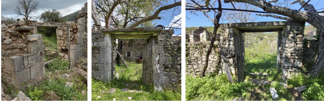
Image 3-38. Courtyard doors made with jambs of stones with carved faces. The upper part of them in the area of the lintel has been replaced with a reinforced concrete slab. Source: NTUA Research Team, 2023.
