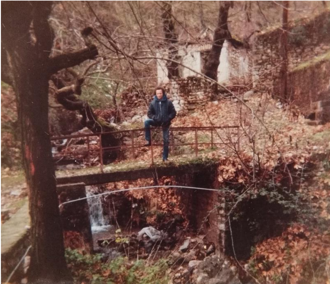
Image 3-46. Characteristic image of the stream from the 1980s. The small bridge, the path, and the ground-floor tavern-grill building upstream of the Vinians fountain are visible. This configuration and the building were completely destroyed in the following years, after a flood that caused embankment failures at a higher point. Photo: Kostas Monias.
