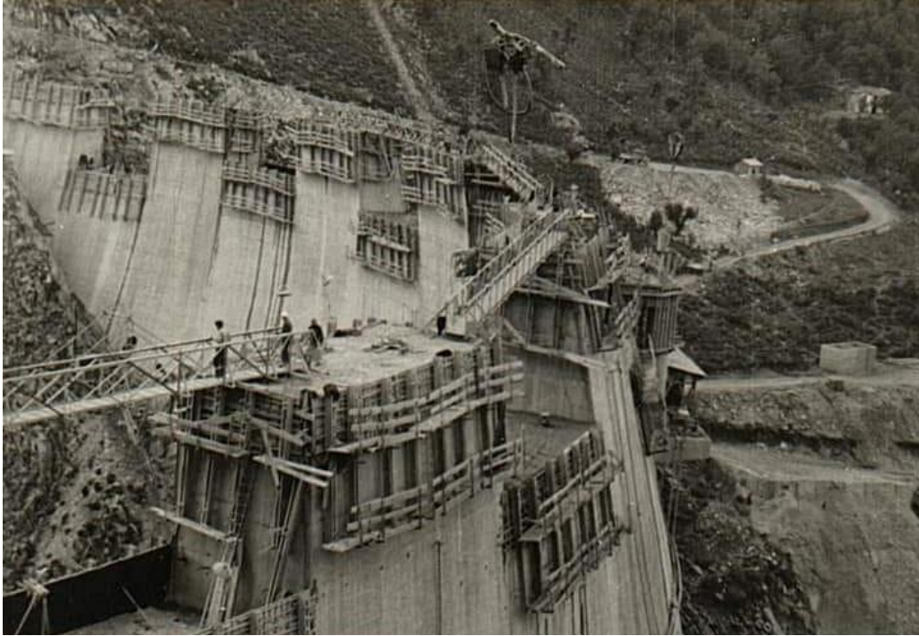
Image 1-31. Construction of Plastiras dam 1959. Source: DEI Photographic Archive.
