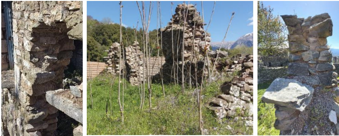
Image 3-29. Three-layer masonry. Source: NTUA Research Team, 2023.
