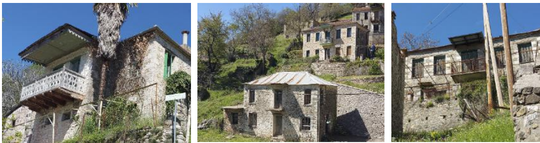
Image 3-44. The best preserved wooden balcony of the House of "Svóllos" (left). Balconies made of reinforced concrete that replaced wooden ones. Source: NTUA Research Team, 2023.
