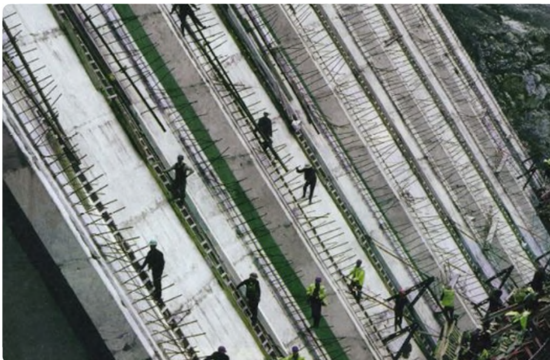
Image 1-32. Construction of the Kremaston dam 1963-1965. Photo: Kostas Balafas. Source: DEI Photographic Archive.
